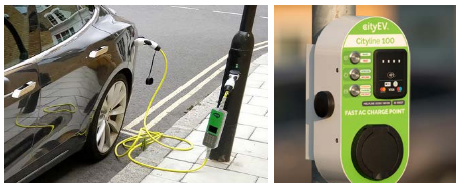
Figure 4 – Lamppost chargepoints of different designs
