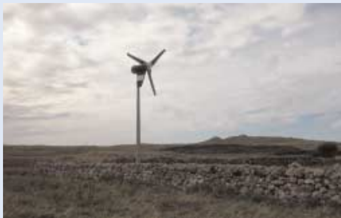
Fig 1: 2.5kW wind turbine used to provide electric storage heating for a household in the Inner Hebrides. Copyright Energy Saving Trust.
