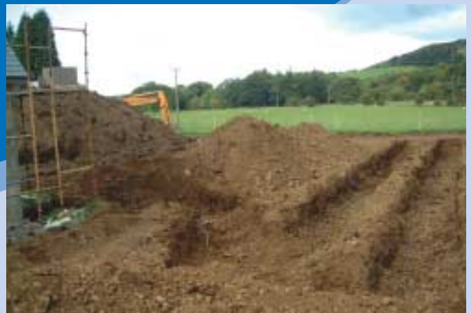
Mr Maxwell's ground loops during installation
