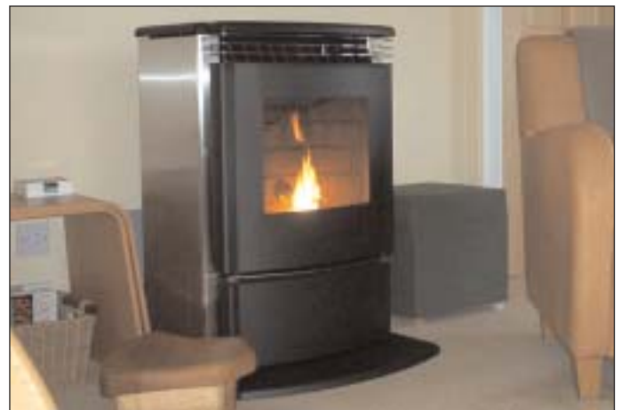
Fig 1: 8.8kW automated pellet stove installed with the help of SCHRI household grant.
