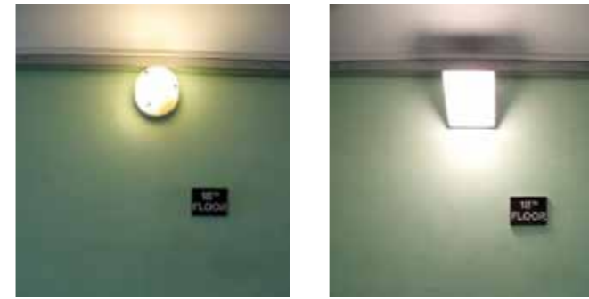
Pre-installation and post-installation
