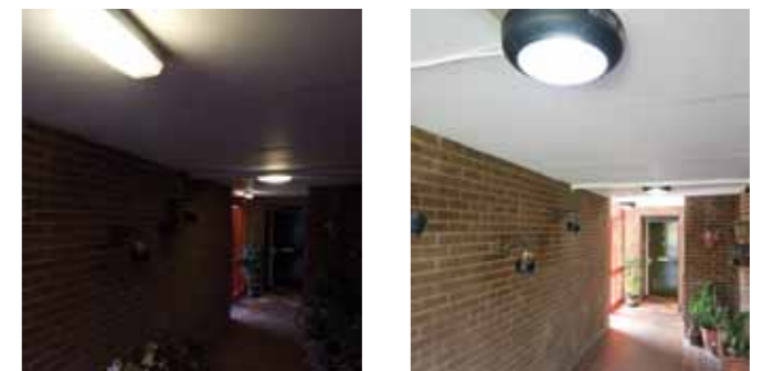
Pre-installation and post-installation
