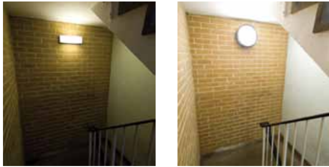
Pre-installation and post-installation
