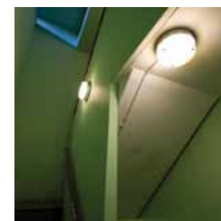
Gambier House (before)
