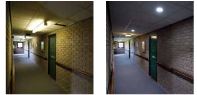
Pre-installation and post-installation
