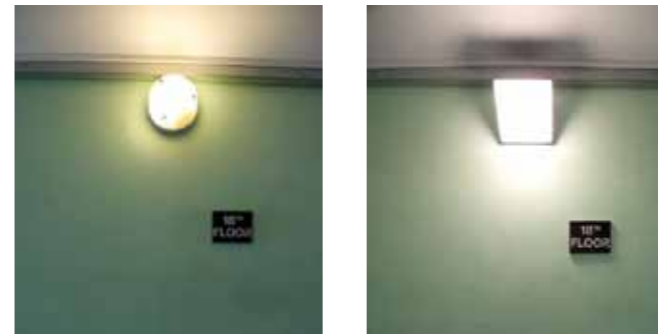
Pre-installation and post-installation
