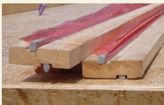
Figure 1 Foam tape is applied to sole plates which expands in place to seal between joints
