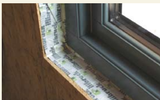
Figure 2 Sealing tape applied to window frame and wall junction
