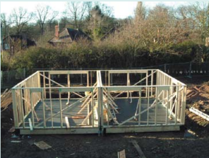
Figure 3 Timber frame construction on site, Glaziers Lane
