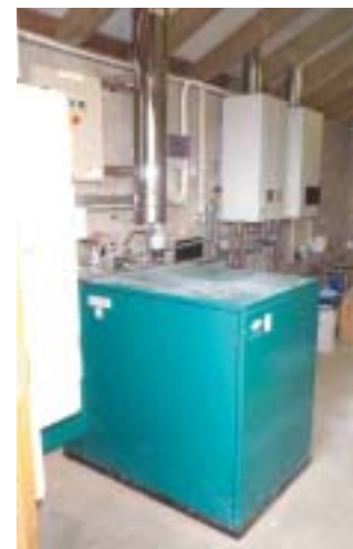
Station Road, Newmachar, Scotland, with energy centre building in foreground and interior view showing the 5.5kW e CHP unit and two wall-hung gas condensing boilers.
